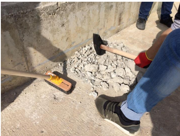
Fig. 2 Crushing demolition rubble manually to obtain sand and fine aggregate
