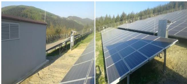
*Fig.2c: The shading of the transformer building is on the Panels*
