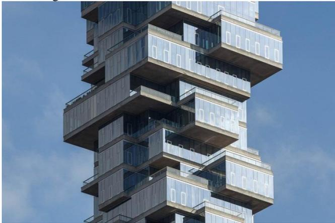
Fig. 8 Strong Concrete Use For Cantilevers of 56 Leonard
