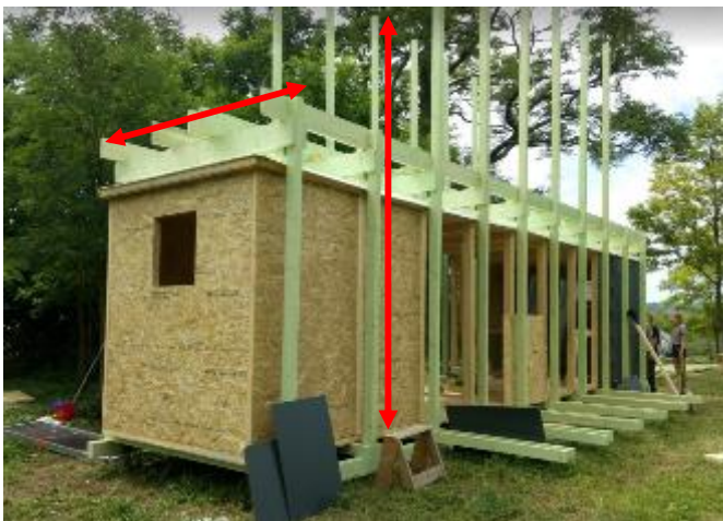
Fig. 23 The installation of outer posts and floor beams for upper floor.
