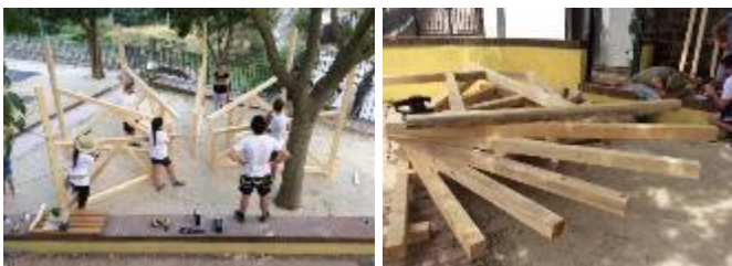
Fig. 12 The heavy trusses stacked and positioning them on site.
