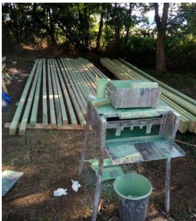
Fig. 27 The wood treatment with green paint on site.
