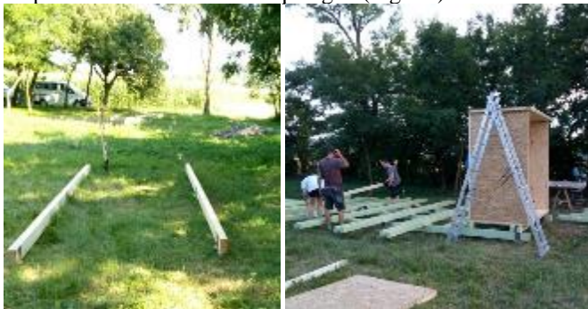
Fig. 19 The base and first installations of the project.
