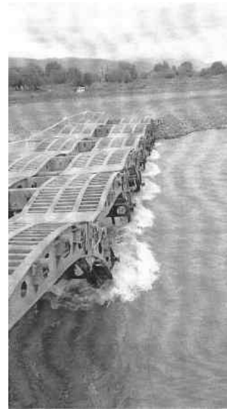
Fig. 7 Multi-span inventory bridge
